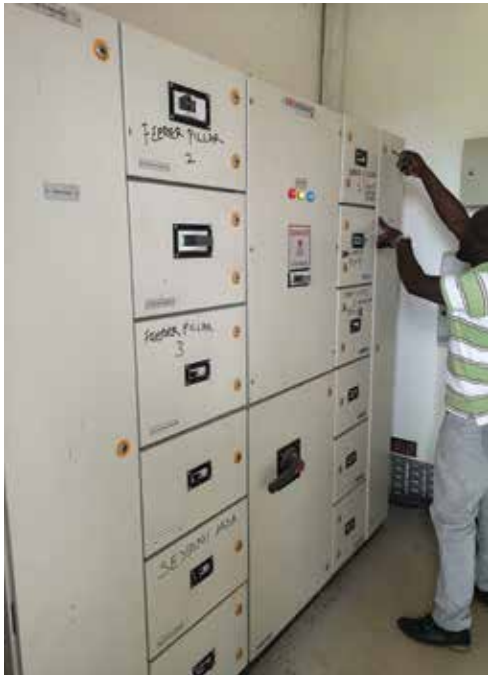
Indoor feeder pillar installation
