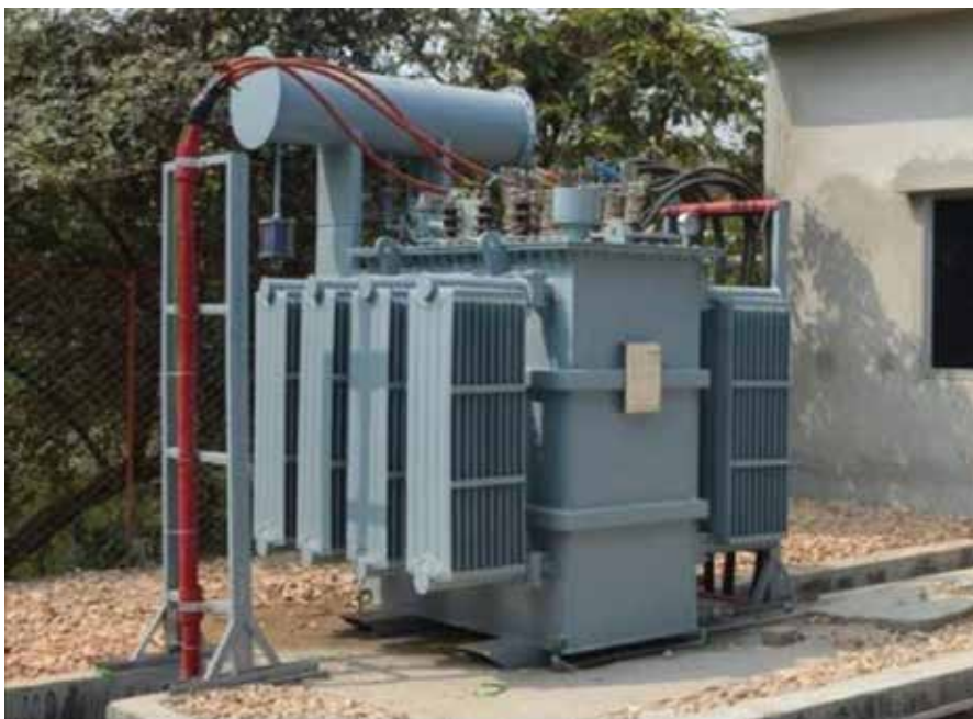
Outdoor ground mounted distribution transformer
